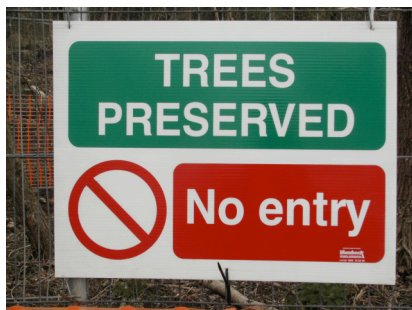
'Protected Tree Zone' signage to be securely attached to the fence
