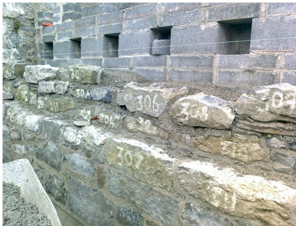
East wall under construction with numbered stones being reinstated exactly in accordance with the survey drawing, and the wall is further advanced below.
