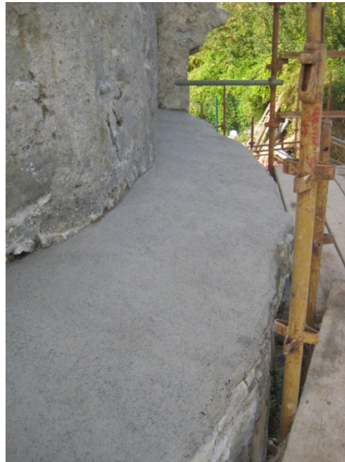
New lime capping to the wall walk
