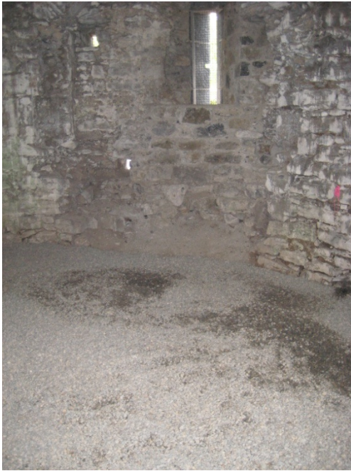
Gravel base to tower interior laid over a geotextile membrane
