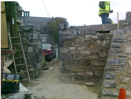
Rebuilding of section of north curtain wall under construction.
