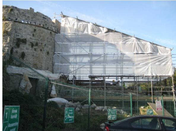
Covered scaffolding allowed for working in inclement weather and protecting the work on completion. Below two corbel stones were reinstated.
