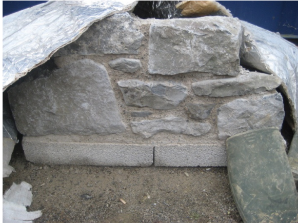
Sample of stonework and mortar approved before works commenced.
