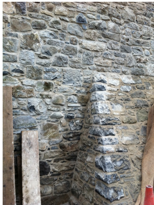
Two views of the corner of the base batter, under construction and completed
