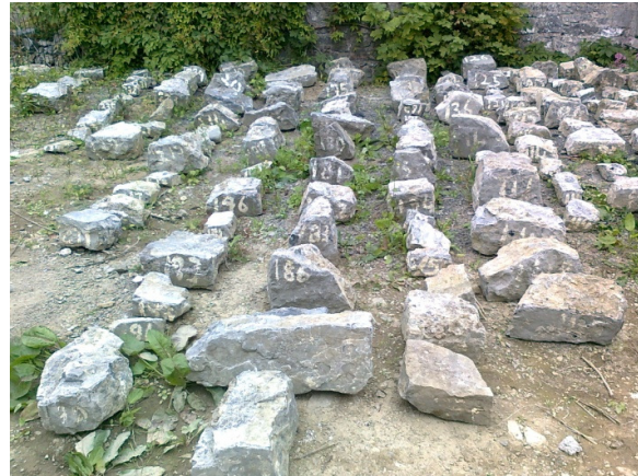
Numbered stones set out in preparation for reinstatement.
