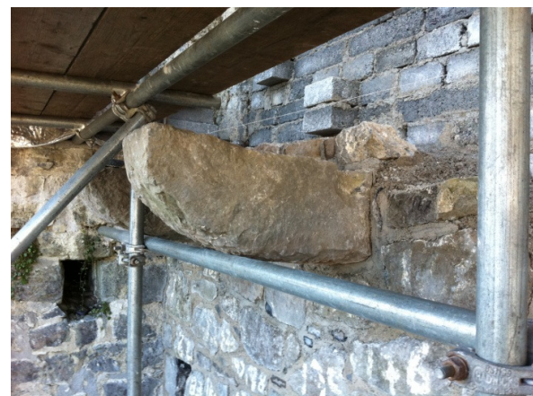
Covered scaffolding allowed for working in inclement weather and protecting the work on completion. Below two corbel stones were reinstated.
