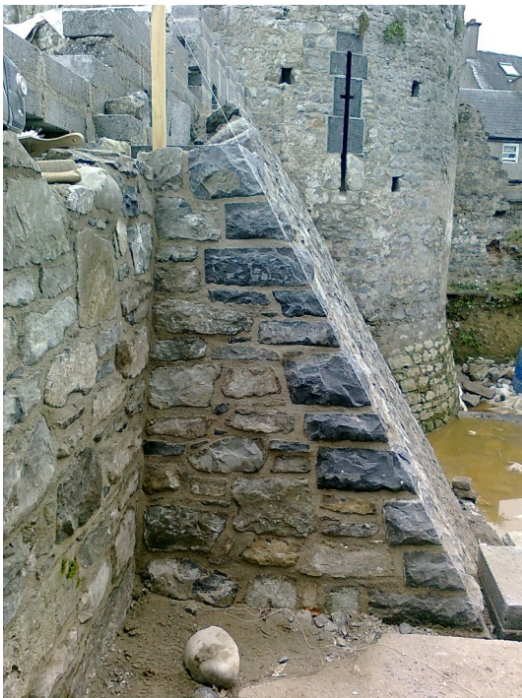
Two views of the corner of the base batter, under construction and completed
