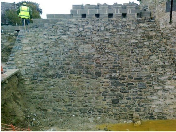
Two views of the base batter repaired and built up to its original height.
