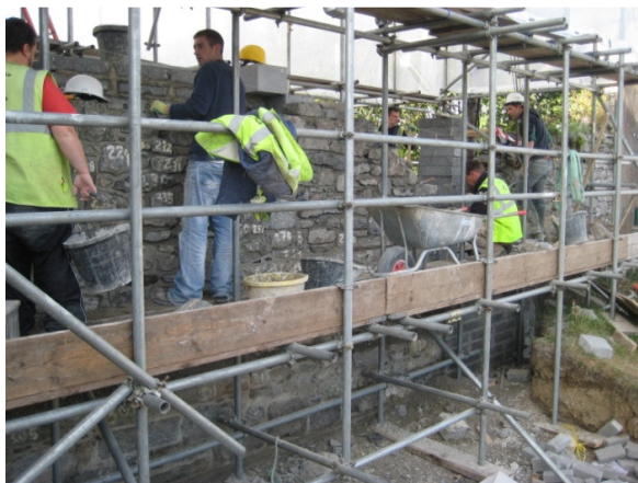
East wall under construction with numbered stones being reinstated exactly in accordance with the survey drawing, and the wall is further advanced below.
