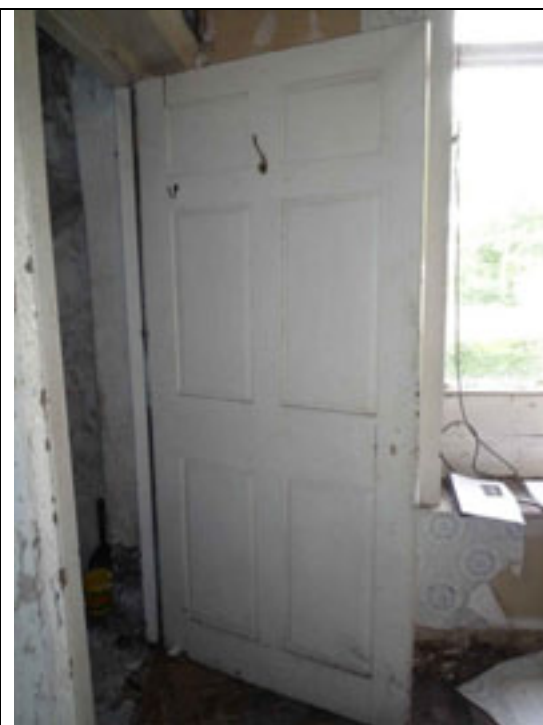
Fig.70: Single-leaf door with raised-and-fielded timber panels giving access to G01.
