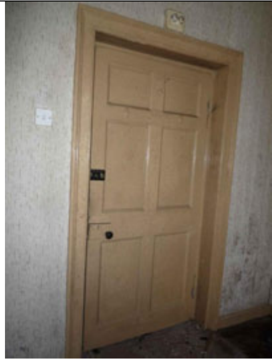
Fig.44: Timber panelled door giving access to G08.
