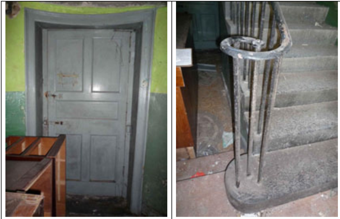
Fig.97: Timber panelled door giving access to the exterior (rear/east). Note the architrave follows the curve of the room.
