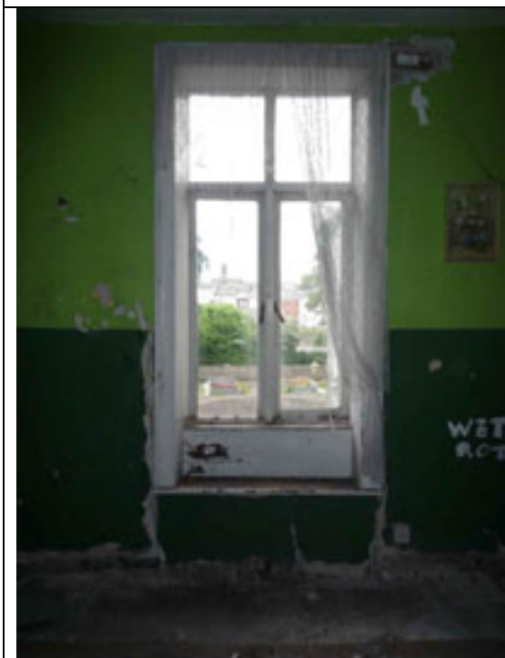
Fig.165: Window opening in the west wall with timber architrave and shutters.
