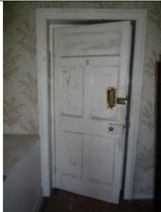
Fig.124: Timber panelled door giving access to G22.
