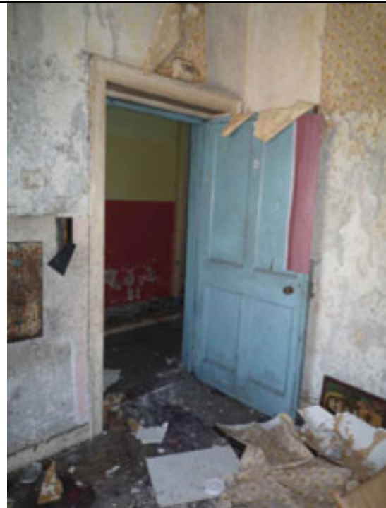
Fig.148: Single-leaf timber panelled door giving access to F08.
