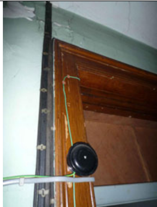
Fig.86: Timber architrave indicating dimensions of original door opening in the north wall.
