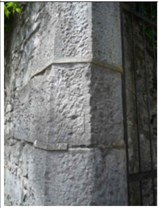
Fig.26: Chamfered limestone surround to archway.
