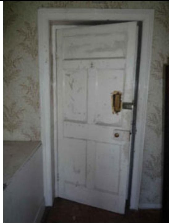
Fig.120: Single-leaf timber panelled door giving access to G22.
