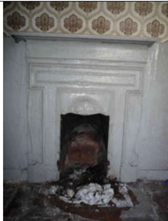
Fig.114: Cast-iron fireplace to west wall.
