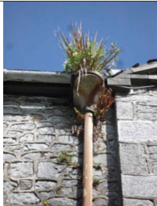
Fig.8: Early-to-mid 20 th century cast-iron hopper head and round downpipe.
