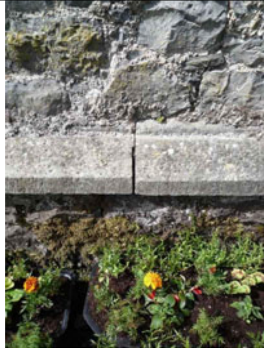
Fig.10: Ashlar plinth course to base of wall - note the exposed rubble limestone walls to remainder.
