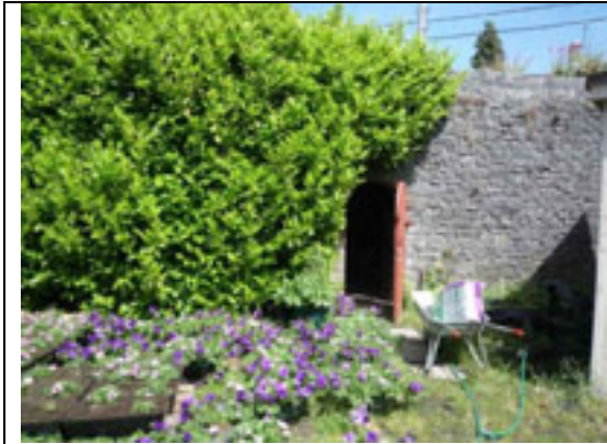
Fig.31: Former sanitary block to the northeast of the site. Note the round-headed door opening.
