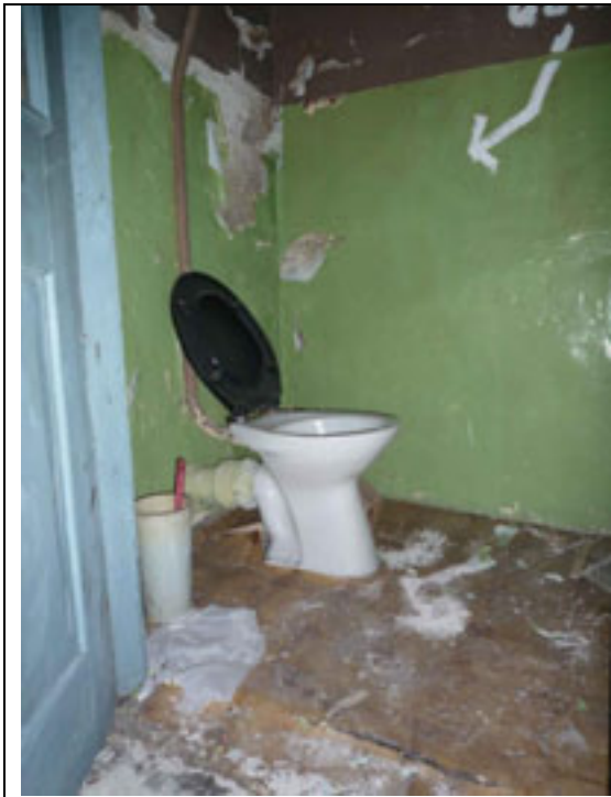
Fig.159: Toilet to G09.
