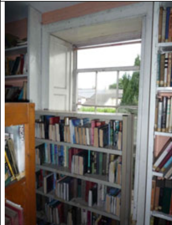
Fig.171: Early timber sliding sash window and associated joinery.
