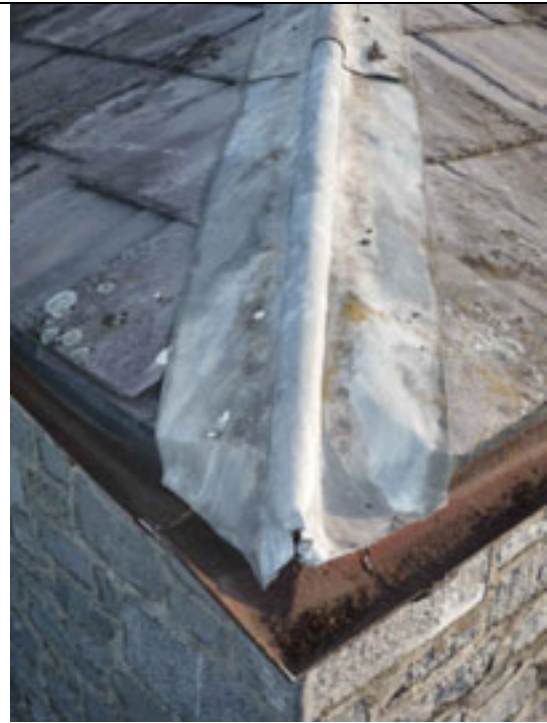
Fig.6: Rolled lead dressed ridge capping.
