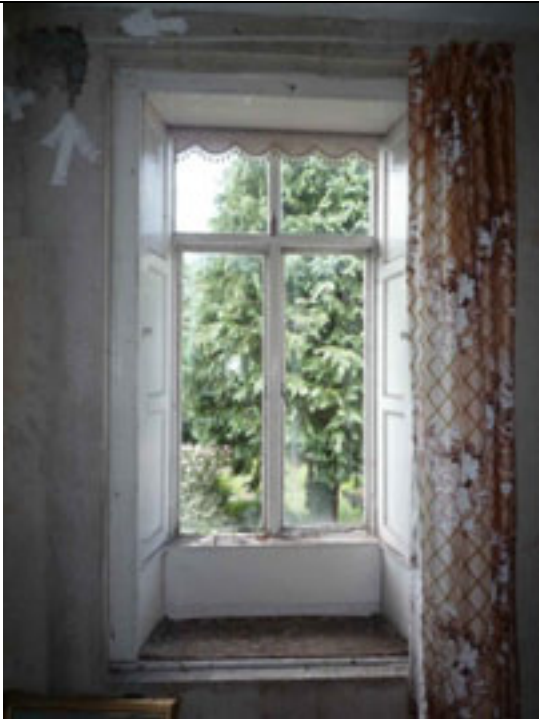
Fig.179: Window opening with early joinery to east wall.
