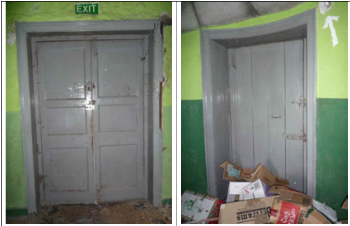
Fig.74: Door giving access to the exterior (rear/east). Note the architrave follow the curve of the room.
