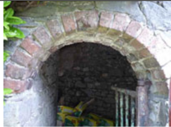
Fig.32: Brick-lined arch giving access to the former sanitary block to the northeast of the site.
