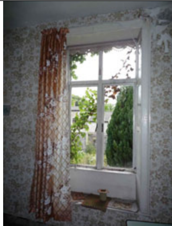
Fig.180: Window opening with early joinery to west wall.
