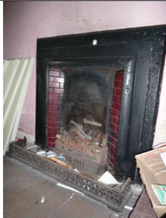
Fig.80: Painted stone fire surround with cast-iron register grate and fender.
