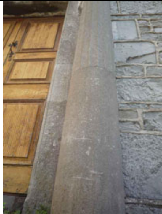
Fig.18: Part fluted engaged Doric column to the principle/west elevation.
