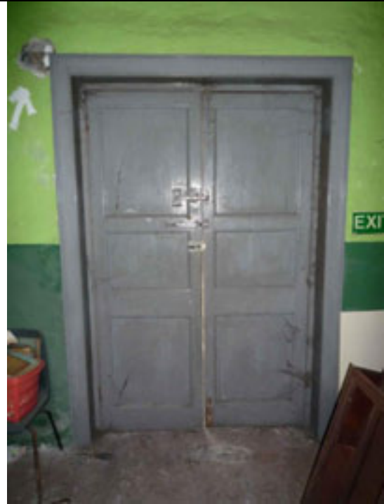
Fig.96: Double-leaf doors giving access to the exterior (front/west).
