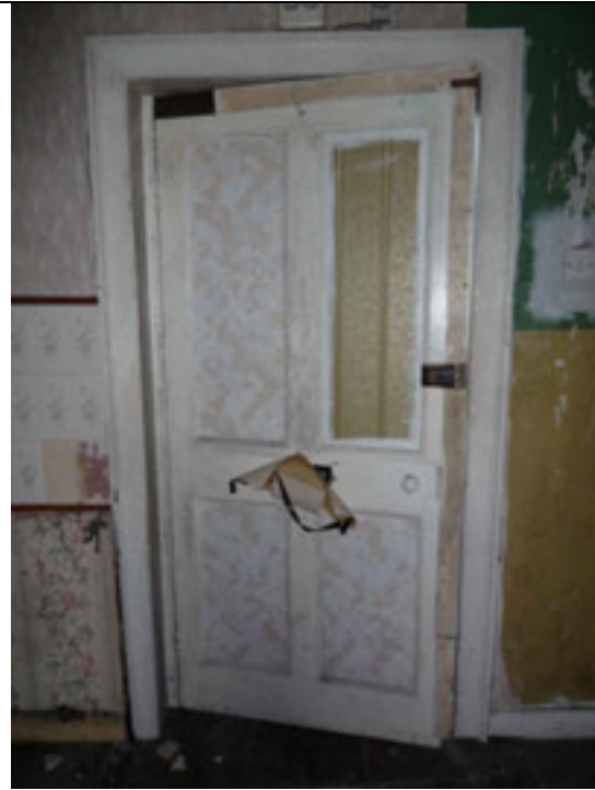
Fig.144: Timber door with four panels giving access to F08.
