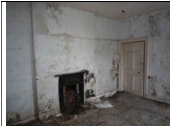
Fig.39: Aspect of room taken from the northwest.
