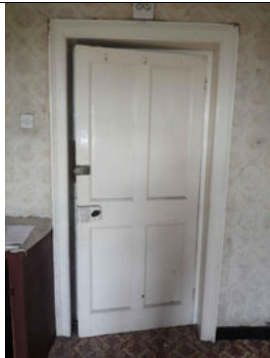
Fig.212: Single-leaf timber panelled door giving access to F21.
