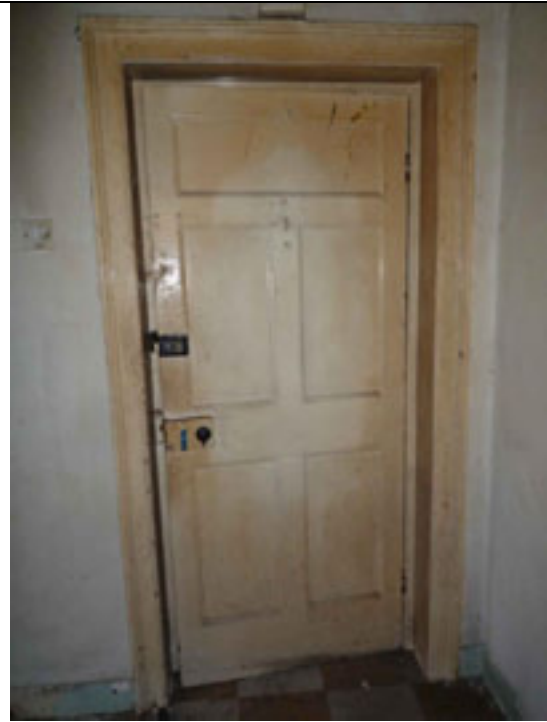
Fig.128: Single-leaf timber panelled door giving access to G22.
