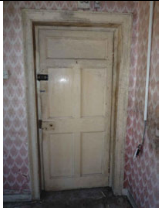
Fig.56: Single-leaf timber panelled door giving access to G08.
