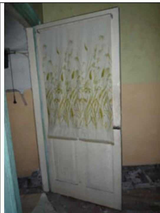
Fig.194: Single-leaf timber panelled door with glazing giving access to F21.
