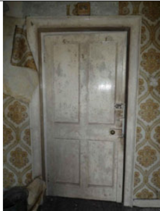
Fig.140: Single-leaf timber panelled door giving access to F08.
