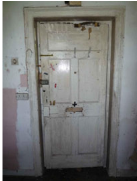
Fig.116: Timber door with five panels giving access to G22.
