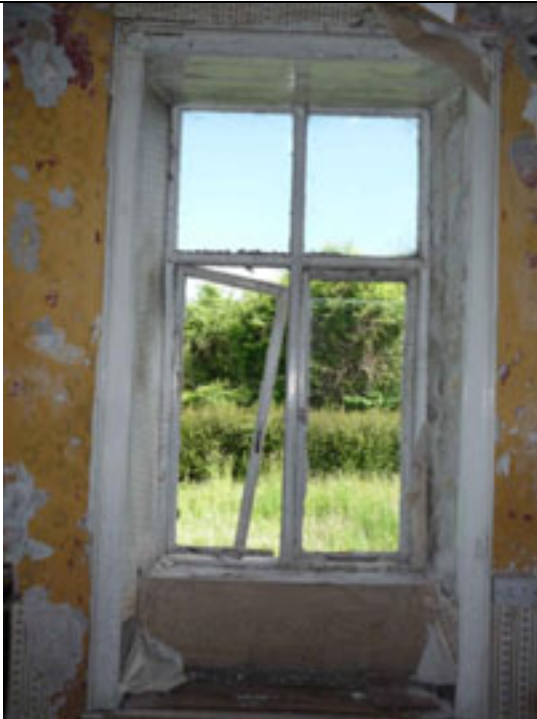
Fig.121: Window opening showing timber architrave.
