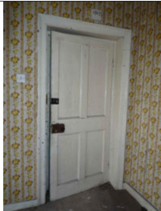
Fig.220: Single-leaf timber panelled door giving access to F21.
