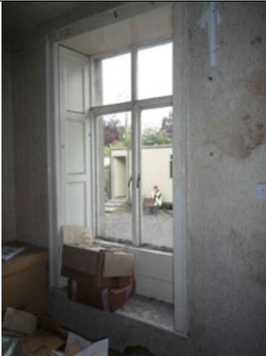
Fig.45: Window opening with surviving timber joinery. Note the replacement casement window.
