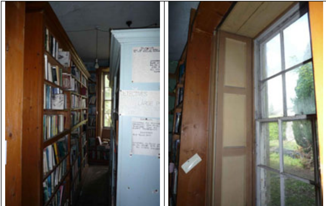
Fig.92: Panelled shutters and early timber sliding sash window.
