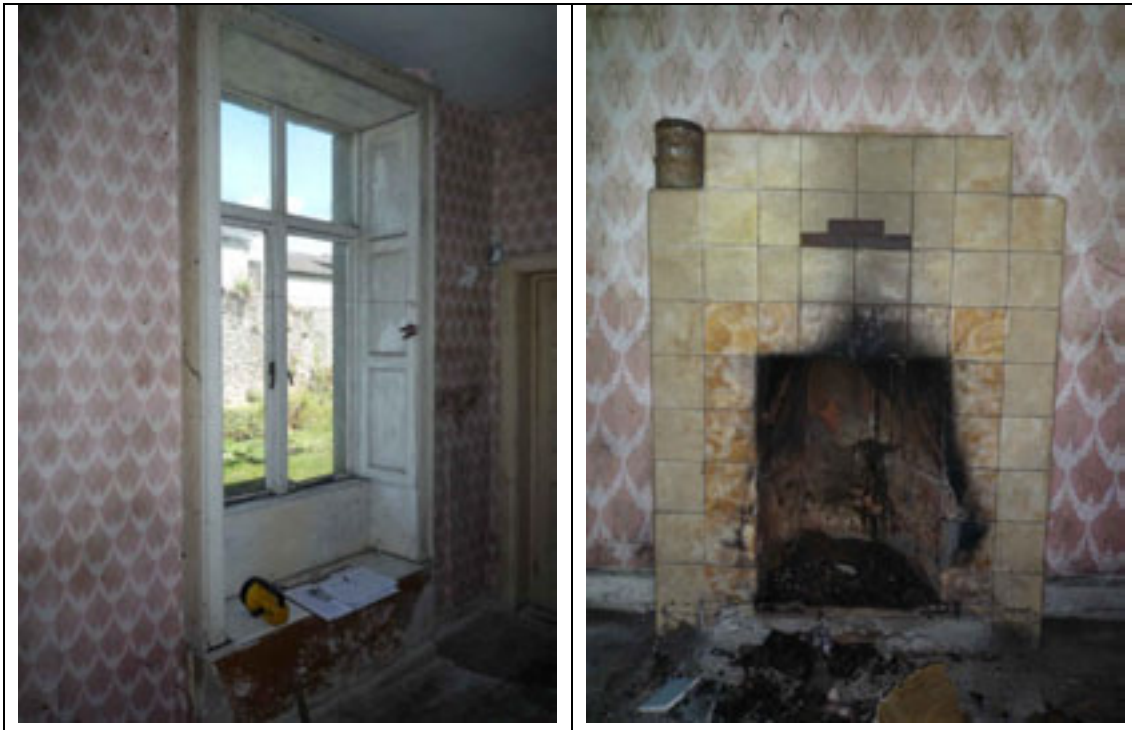
Fig.57: Early timber window joinery. Note the architrave rests on a projecting window apron.
