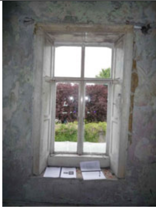
Fig.141: Window opening showing timber panelled shutters.
