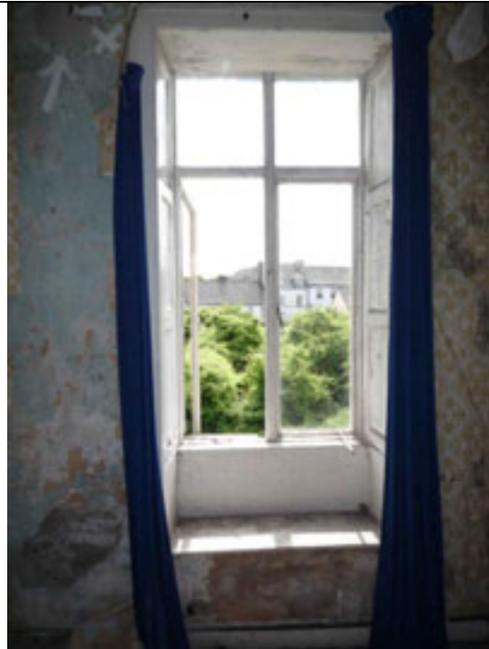
Fig.210: Window opening with surviving timber joinery.
