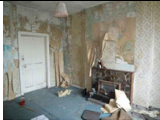
Fig.207: Aspect of room taken from the southwest.
