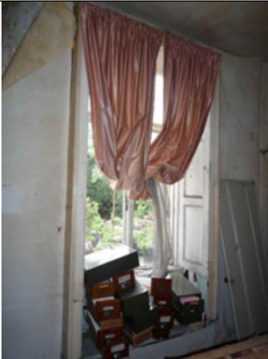
Fig.129: Window opening with surviving timber joinery. Note the replacement casement window.
