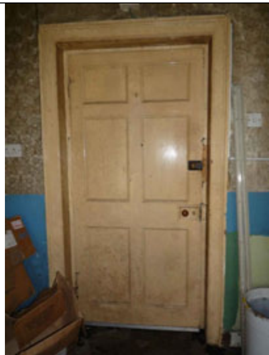
Fig.48: Single-leaf timber panelled door giving access to G08.
