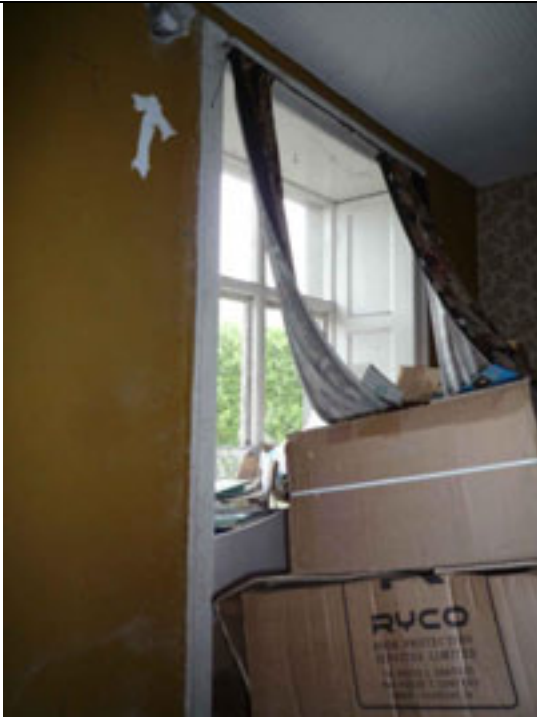
Fig.53: Window opening with surviving timber joinery.
