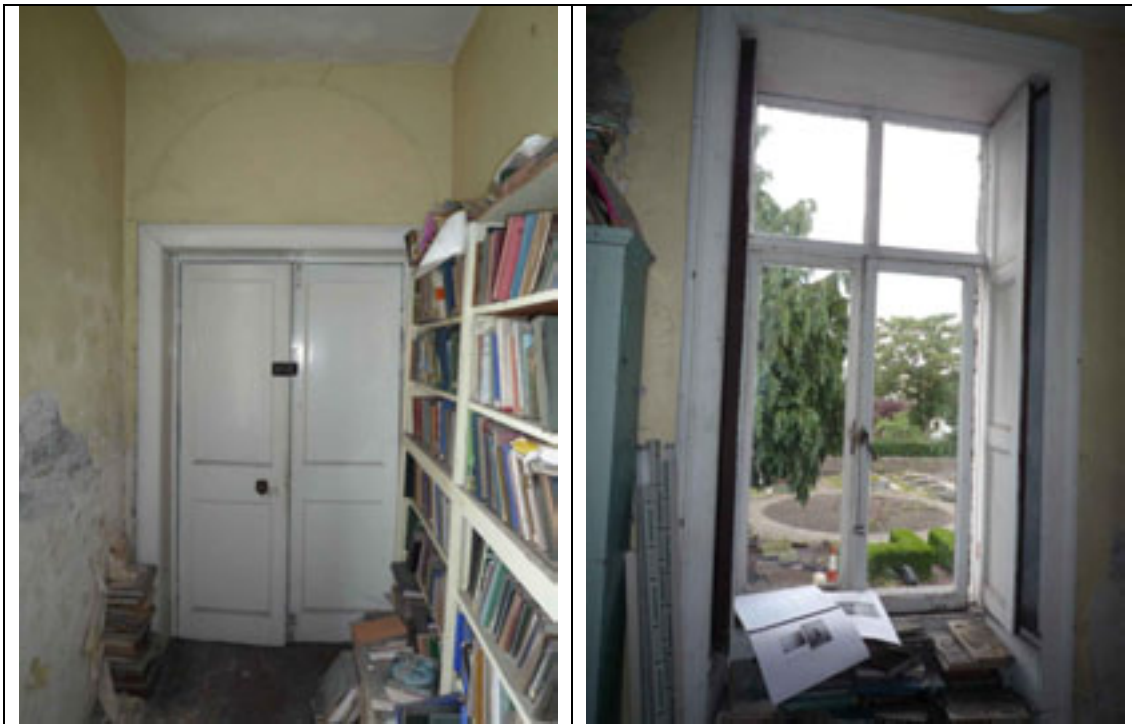
Fig.167: Aspect of corridor taken from the south.
