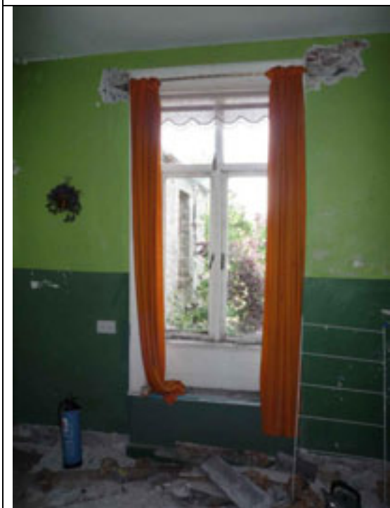
Fig.189: Window opening in the west wall with timber architrave and shutters.
