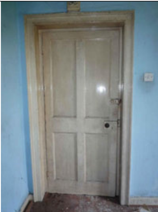
Fig.205: Single-leaf timber panelled door giving access to F21.
