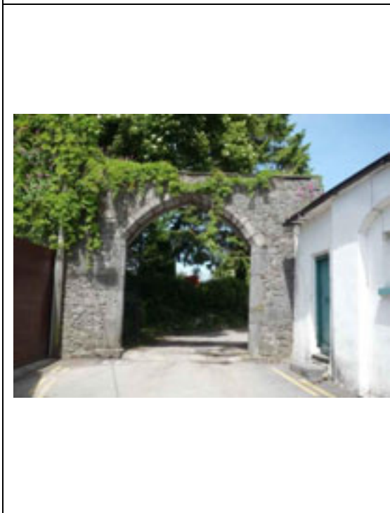
Fig.25: Gateway giving access from Barrack Lane.
