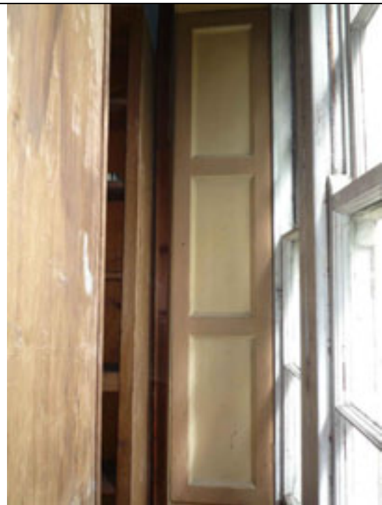
Fig.88: Early window joinery to the wyatt window to the east wall.
