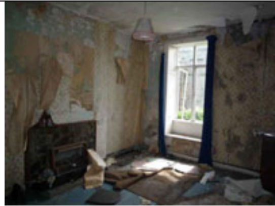
Fig.208: Aspect of room taken from the northwest.
