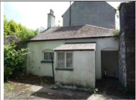
Fig.24: North elevation of gate lodge showing projecting porch.
