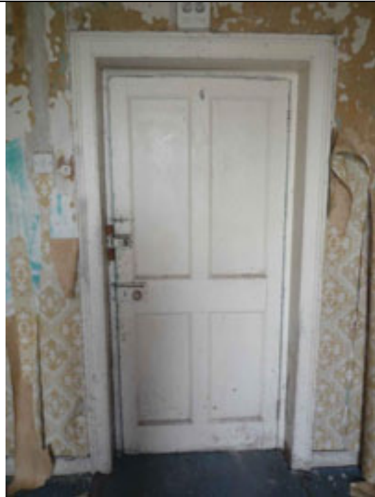
Fig.209: Timber door with five panels giving access to F21.
