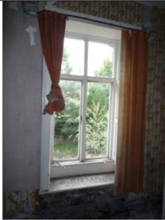
Fig.221: Window opening with surviving timber joinery. Note the replacement casement window.
