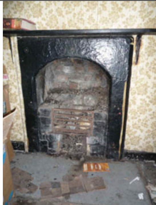
Fig.54: Painted stone fireplace with timber mantel shelf and hob grate.
