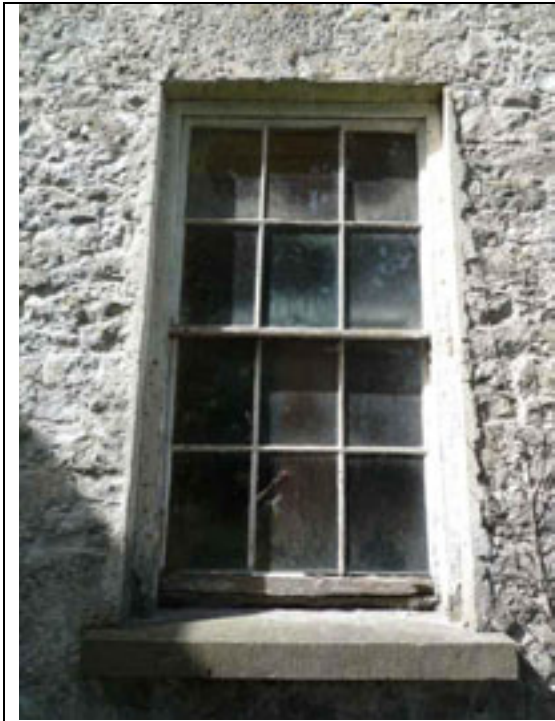
Fig.13: Early timber six-over-six sash window to the east elevation.
