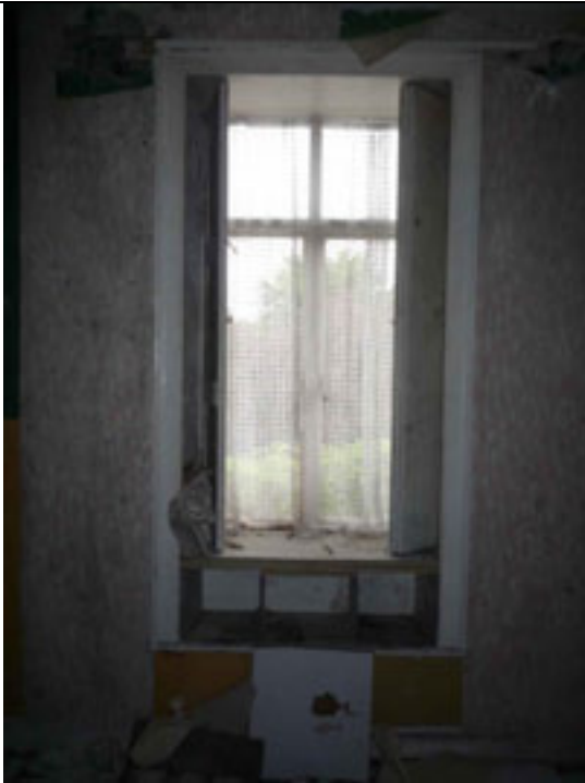
Fig.145: Window opening with surviving timber shutters.
