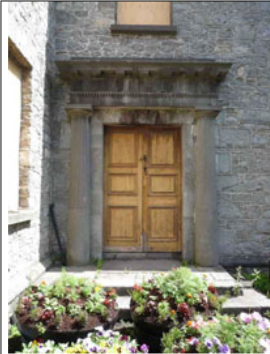
Fig.17: Greek revival doorcase to principle/west elevation.
