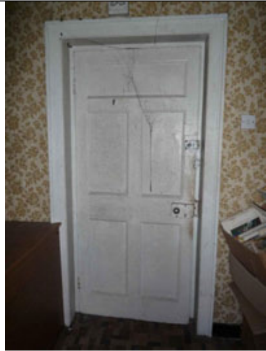
Fig.52: Timber door with five panels giving access to G08.
