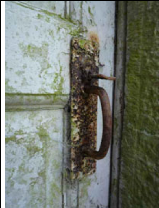
Fig.21: Early thumb-latch to rear/east elevation.
