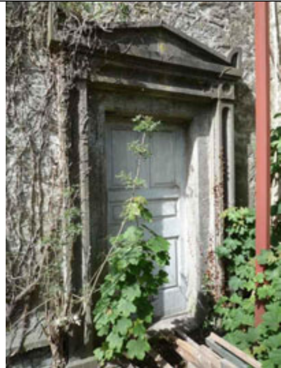
Fig.20: Doorcase to rear/east elevation. Note the raised-and-fielded panelled door.
