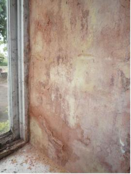
Fig.28: Failure of the plaster to the east window opening.
