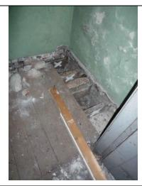
Fig.66: Missing floorboards, timber skirting and failed plaster to room F07.
