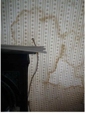
Fig. 50: Soot staining to chimney breast associated with penetrating damp.
