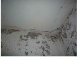
Fig. 19: Failed plaster to the west wall.
