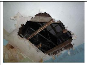
Fig.56: Hole in ceiling plasterwork to the southeast.
