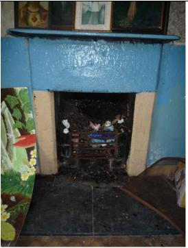
Fig.5: Salts/efflorescence at low level to wall - a visible sign of rising damp.
