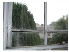
Fig.76: Timber decay to glazing bar of window - note the glass pane has slipped.
