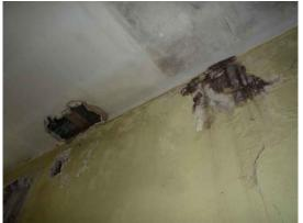
Fig.89: Missing timber floorboards to the north wall.
