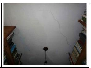
Fig. 31: Cracking of ceiling plaster.
