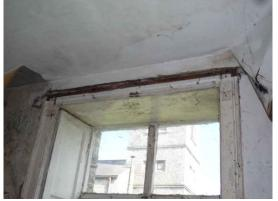
Fig.48: Missing section of architrave to window opening.
