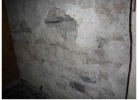
Fig.71: Failed plaster to the west wall.
