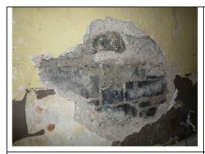
Fig. 15: Missing plaster to the south wall.
