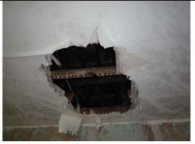
Fig. 102: Hole to ceiling plaster.
