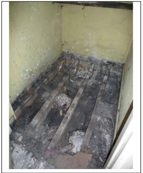
Fig.65: Missing floorboards to F06
