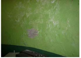
Fig.36: Timber decay to timber skirting to east wall.
