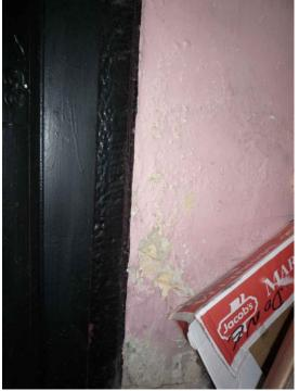
Fig.25: Plaster failure to the east wall indicating rising damp.
