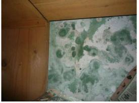
Fig.33: Plaster failure and efflorescence at junction of south and east wall.
