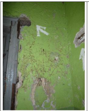
Fig.21: Failure of plaster to the west likely to have been caused by the ingress of moisture through open-joints in the external door surround.
