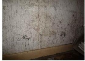
Fig.3: Timber decay to skirting board (north wall).
