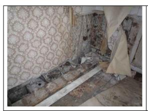
Fig.101: Missing timber floorboards to the east wall.
