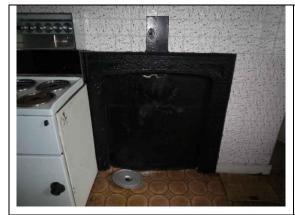
Fig.84: Over-painted stone fireplace with blocked opening.
