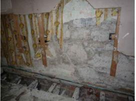
Fig. 103: Missing floorboards to west wall.
