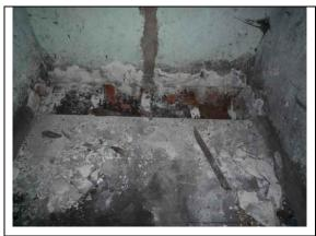
Fig. 93: Missing floorboards to the north wall.
