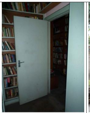
Fig.27: Partially blocked opening to the south wall. Note the inappropriate flush panelled door.
