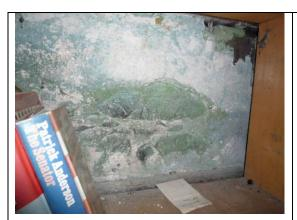
Fig. 32: Plaster failure and efflorescence to east wall.
