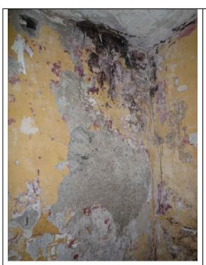
Fig.49: Plaster failure and fungal growth to the east wall.
