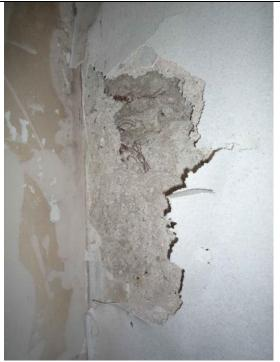
Fig.2: Delamination of wall plaster likely to have been caused by application of cement based pointing to the external elevation.
