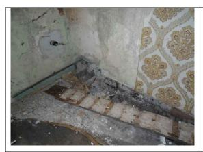
Fig.59: Missing floorboards to the east elevation.
