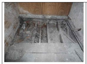
Fig.70: Missing floorboards to the south of room F10.
