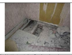
Fig.61: Missing timber floorboards to the northwest corner.
