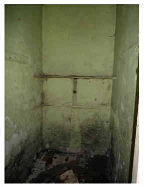
Fig.38: Plaster failure to low level as a result of rising damp.
