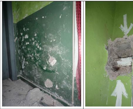
Fig.82: Failure of plaster to the west wall.
