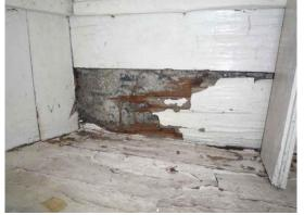
Fig.16: Timber decay to window back of westernmost window opening.
