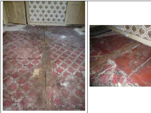
Fig.45: Linoleum floor covering to the limestone flags.
