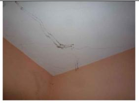
Fig.77: Cracking of ceiling plaster to the southwest corner.
