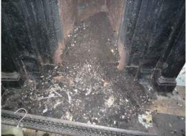
Fig.53: Plaster failure to the west wall of G29.
