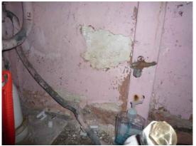
Fig.34: Blocked former door opening in the south wall.
