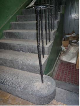
Fig.22: Missing wrought-iron balusters newel post of staircase.
