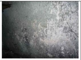
Fig. 94: Penetrating damp to the east wall.
